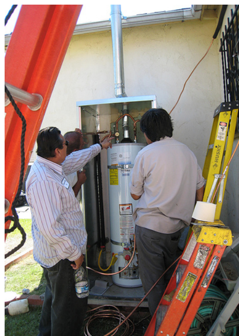
New 40 gallon tank and enclosure after installation.
